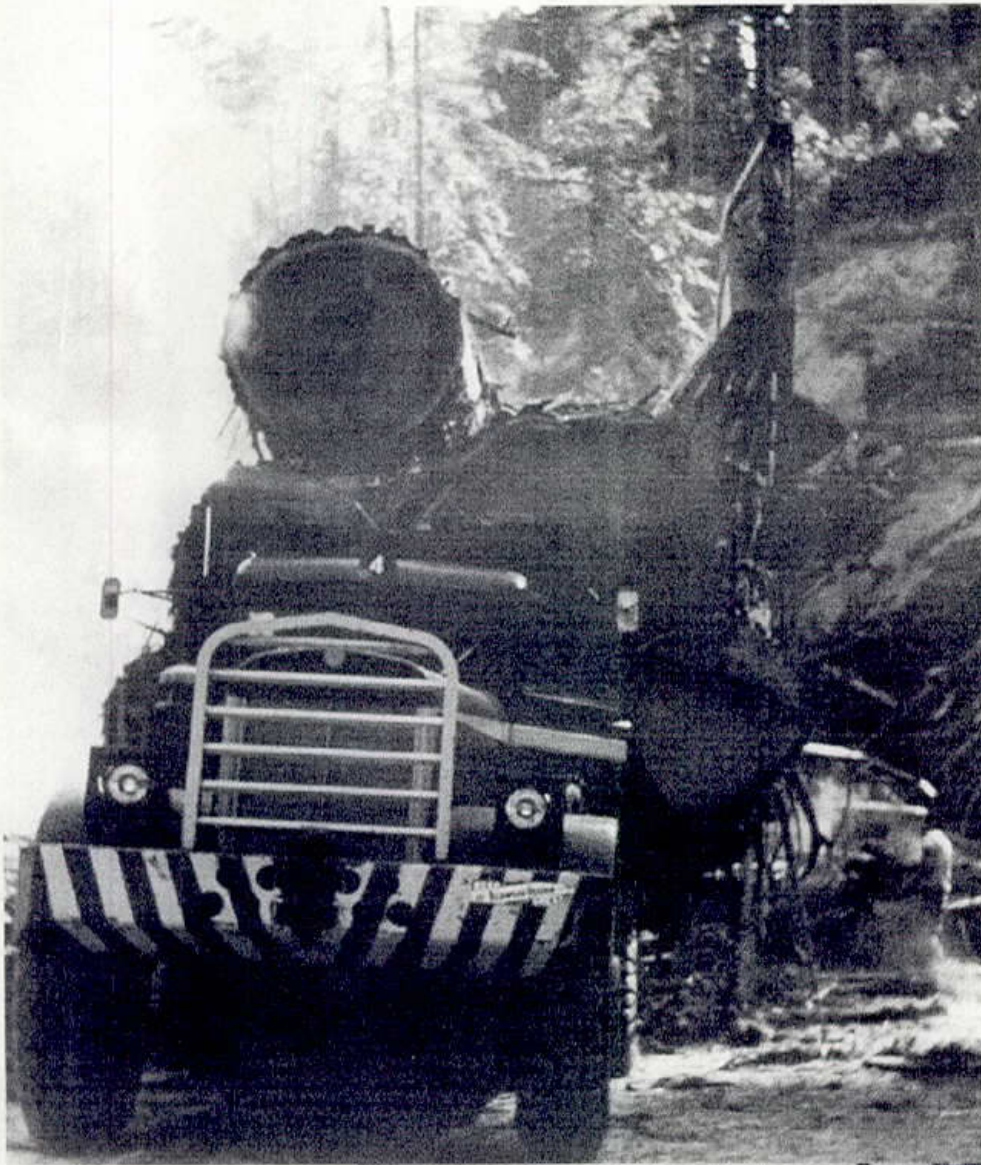
ULCO off-highway truck #4, once Rossi #20, loads under a TL-15 Washington Trak-loader with an International TD-24 on the landing.
